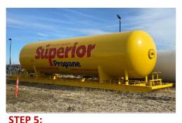
Open liquid valves on opposite end of tank from vapour connection. Ensure air is coming out of liquid ports.
